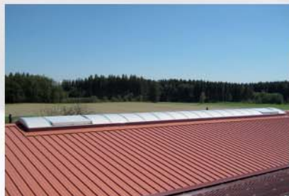
On top of a saddle roof ridge
