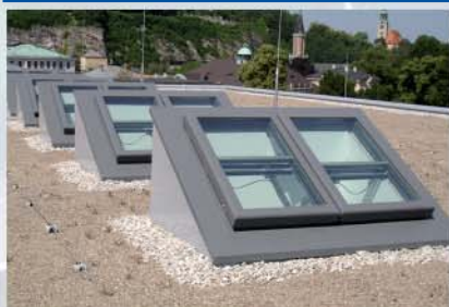
Mounted on a sloped plinth
