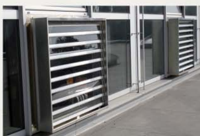
SMOKEJET in vertical glazing
